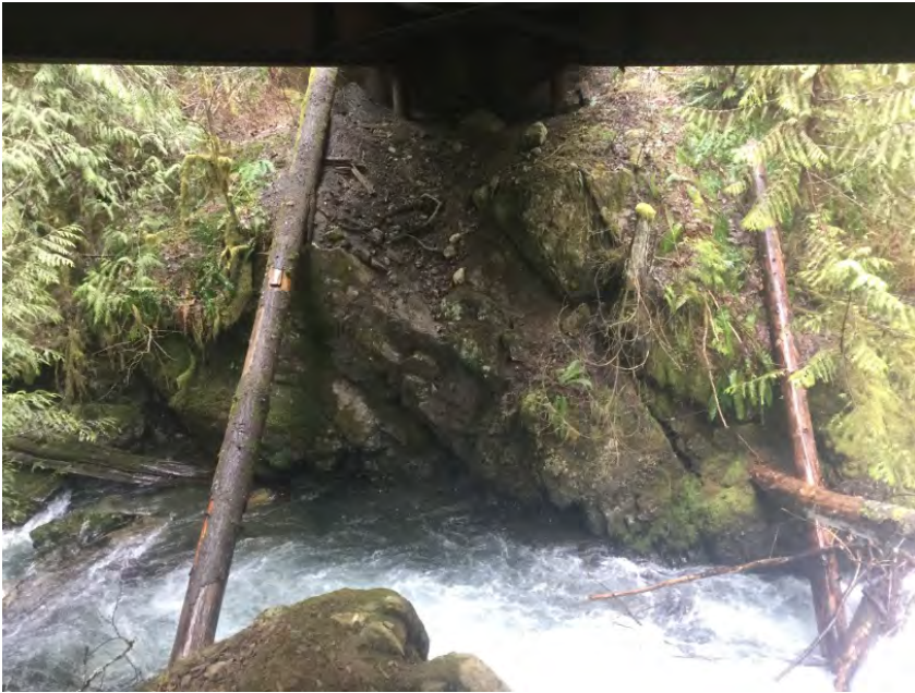
Right Bank Abutment when facing downstream
