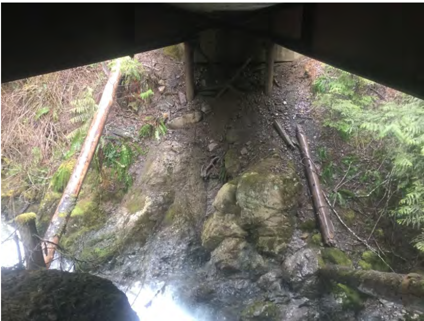
Left Bank Abutment when facing downstream
